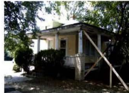
5 HOUSE AT 6924 WILLOW STREET TO BE RELOCATED
