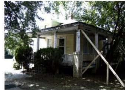
5 HOUSE AT 6924 WILLOW STREET TO BE RELOCATED
