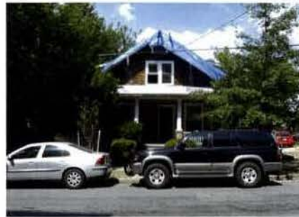
4 HOUSE AT 6926 WILLOW STREET TO BE RELOCATED
