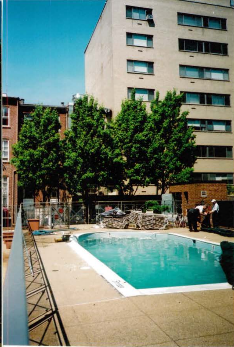
Photo 5 Richmond Pool w/ vent hood above adjacent residences
