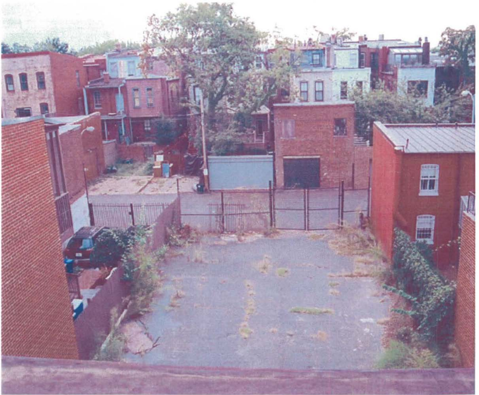
LOOKING FROM ROOF TO REAR
