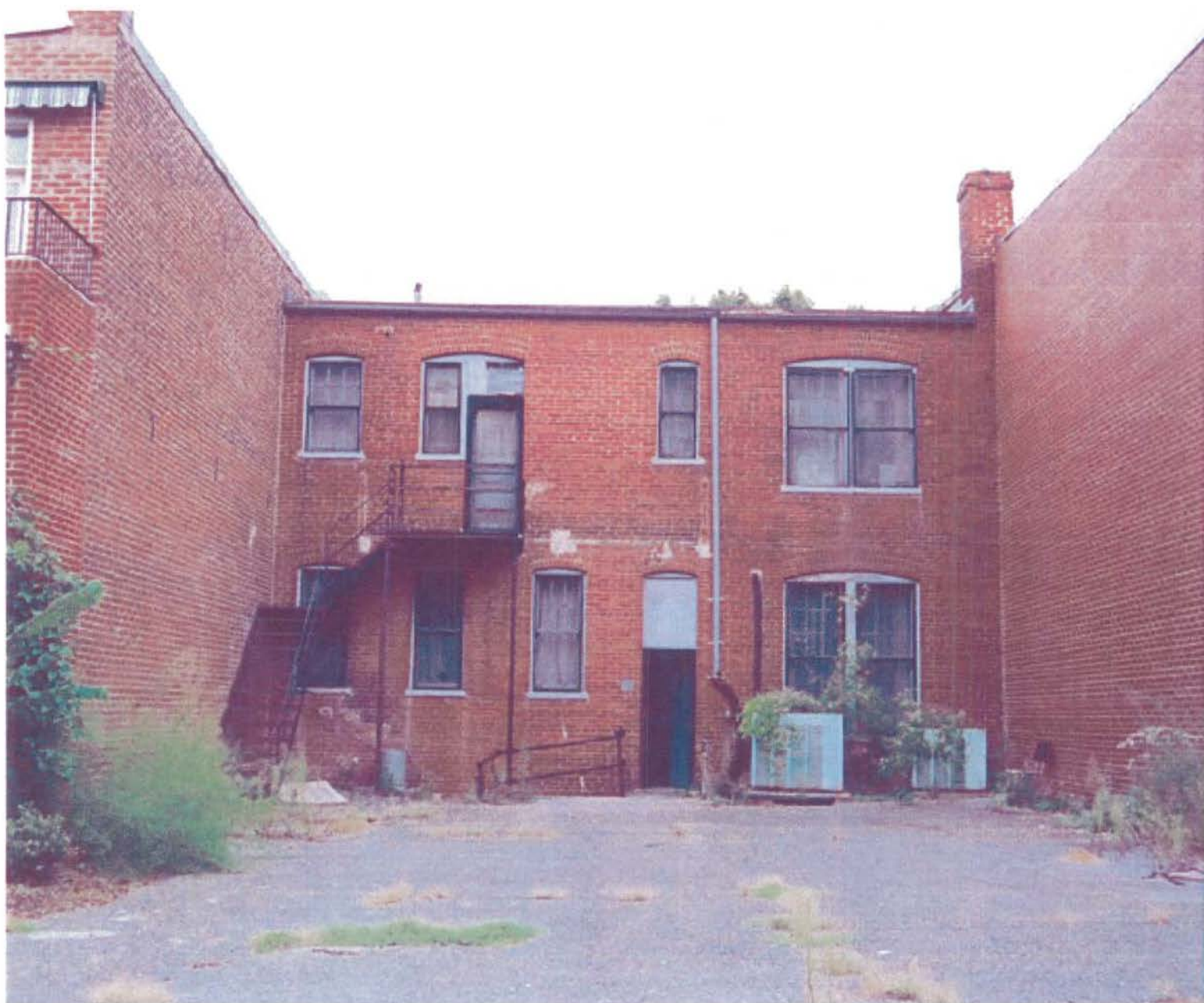
LOOKING AT REAR OF BUILDING
