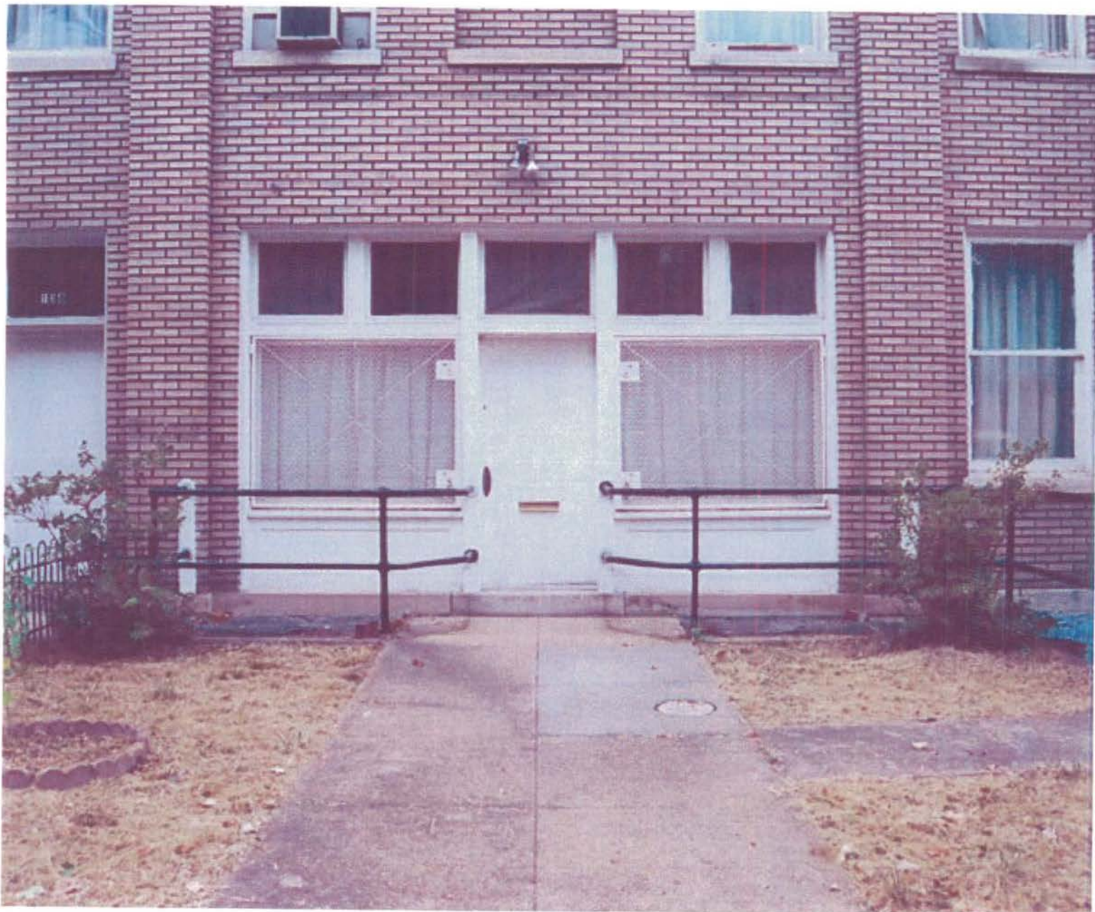
CLOSE UP OF EXISTING ENTRY
