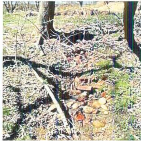
Erosion channel at the NPS property
