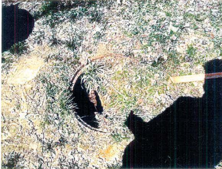
Vent pipe opening for septic tank
