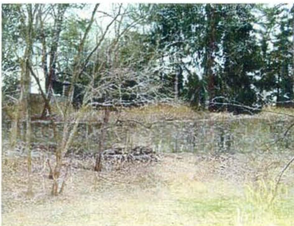
Retaining wall for the former Brady Estate Mansion
