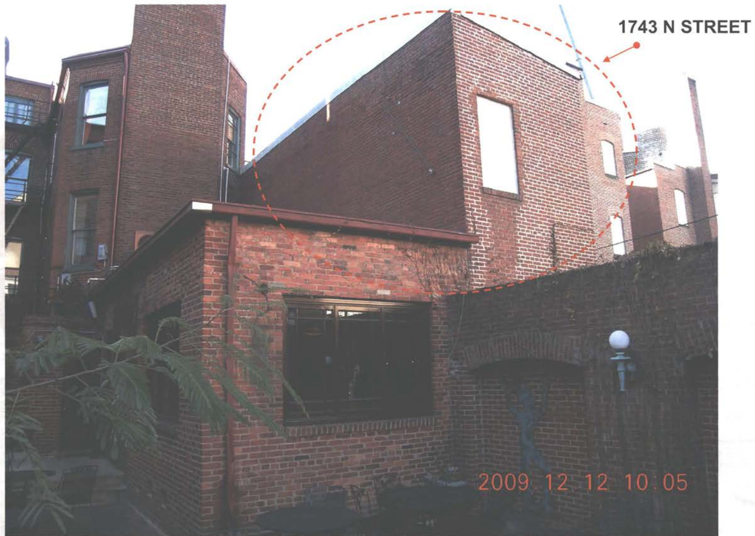
PROPOSED DEMOLITION OF REAR ELL AT 1743 N STREET
