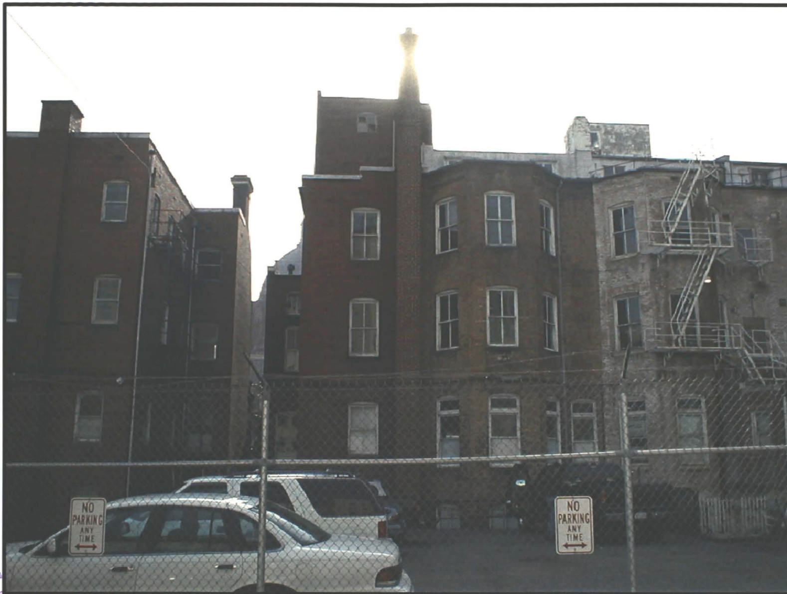
ALLEY VIEW 1745, 1751, AND 1755 N STREET, N.W.
