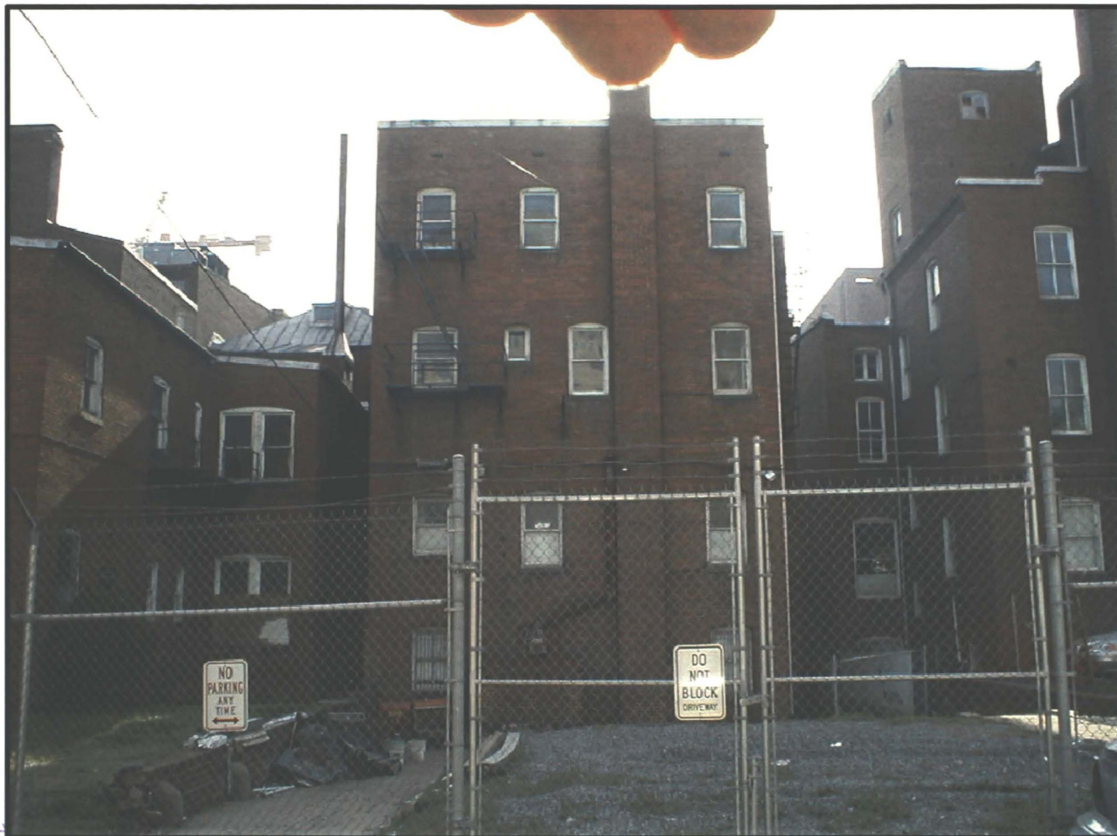
ALLEY VIEW 1743 AND 1745 N STREET, N.W.
