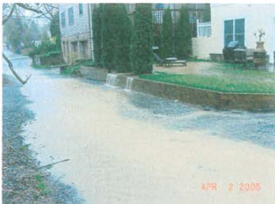
Infiltration trench backs up into 5528's yard and spills over into alley
