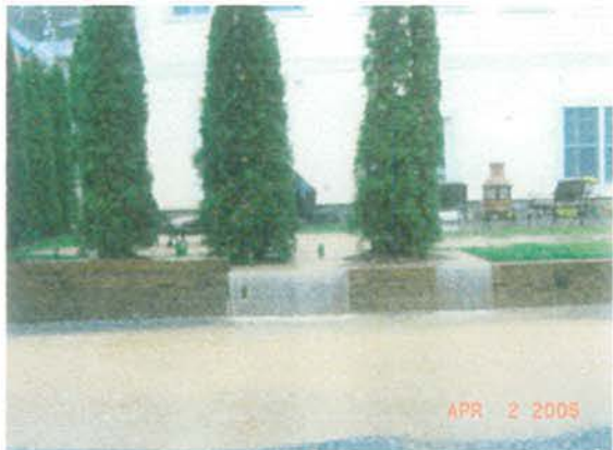
5526/5528 MacArthur's stormwater mgmt system fails
