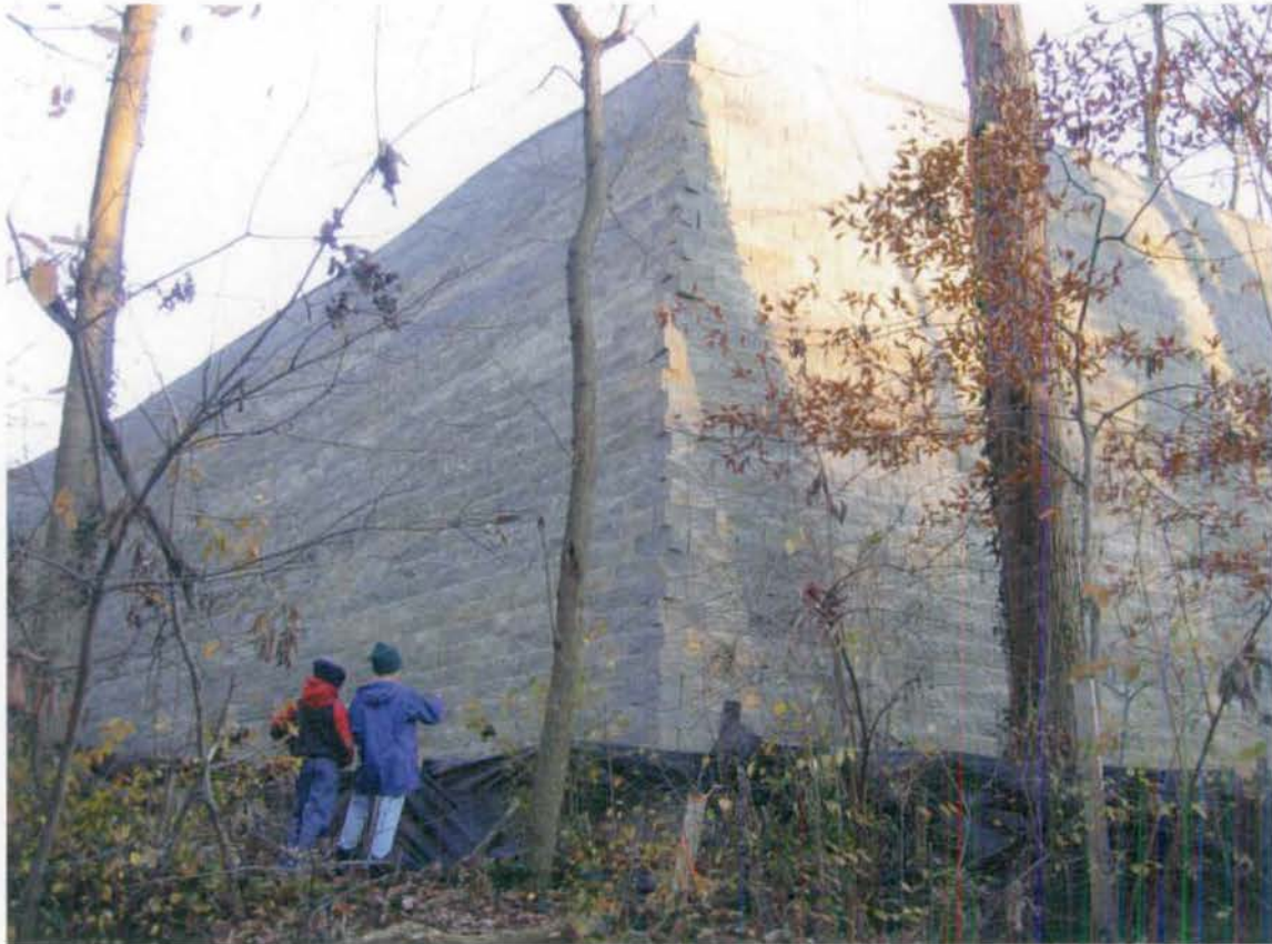
Illustration No 1. (Northwest Corner of Exterior of Illegal Warehouse-Platform Building, 11/28/2004)
