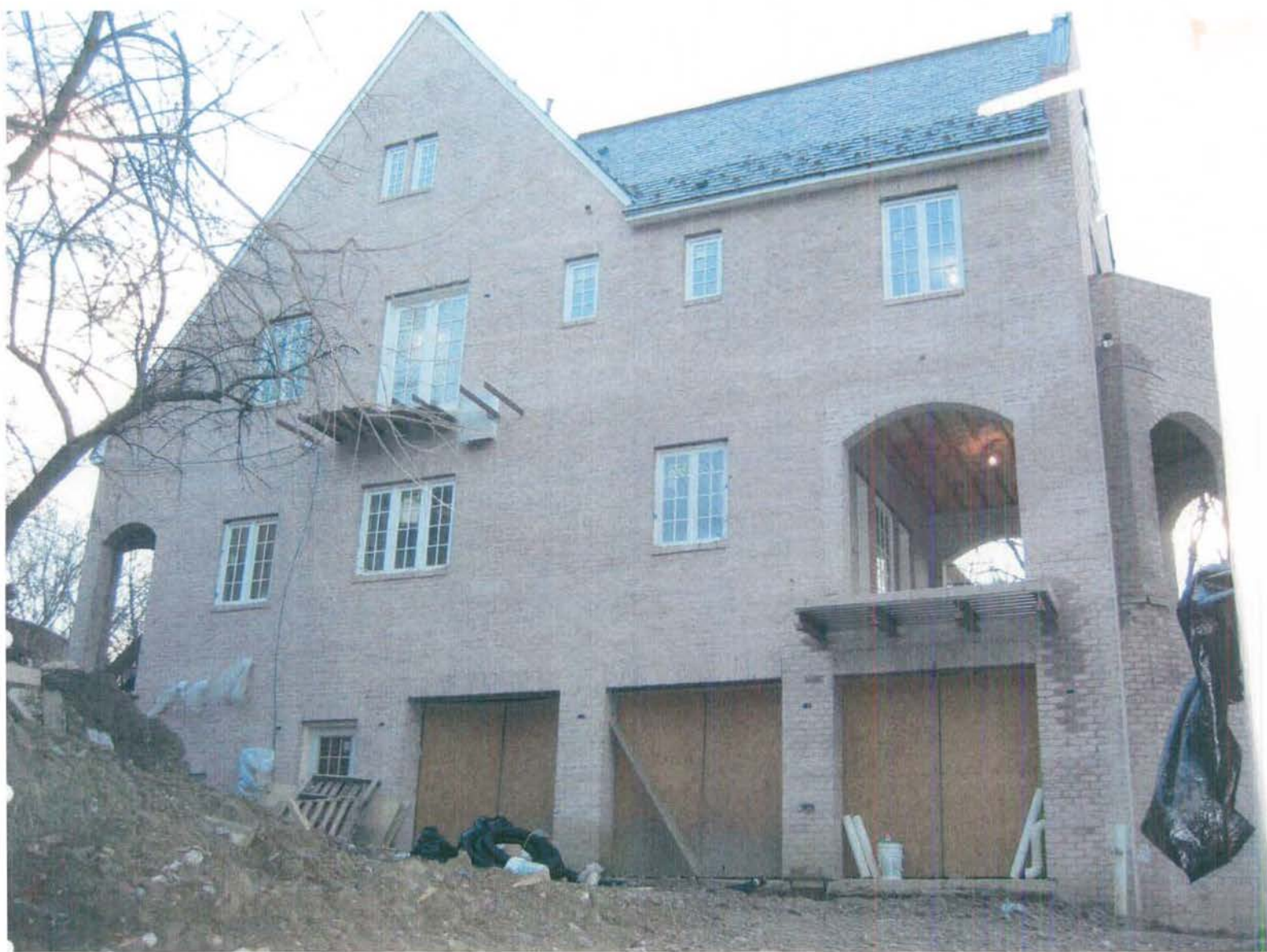
View of new house from its east side
