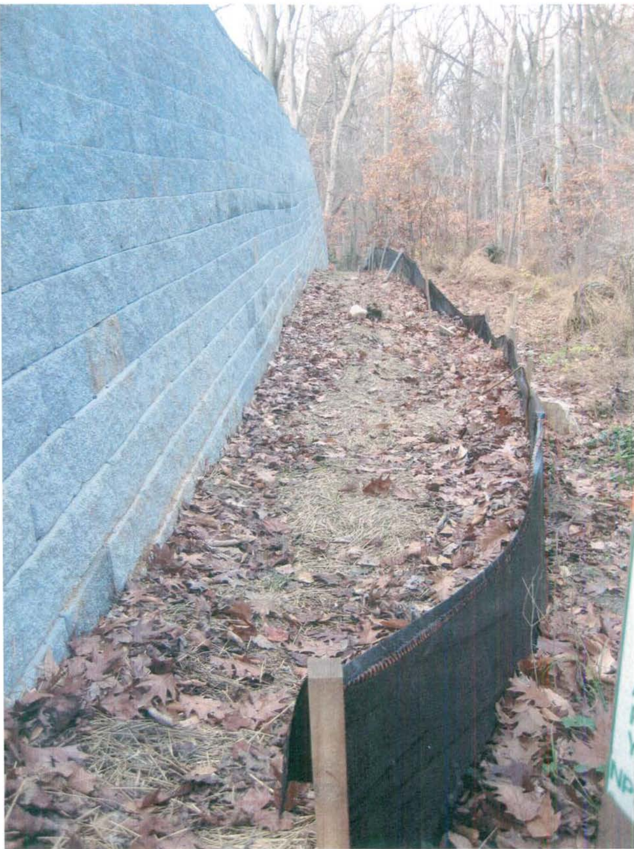
Silt fence located on NPS/Wesley Heights Park Property
