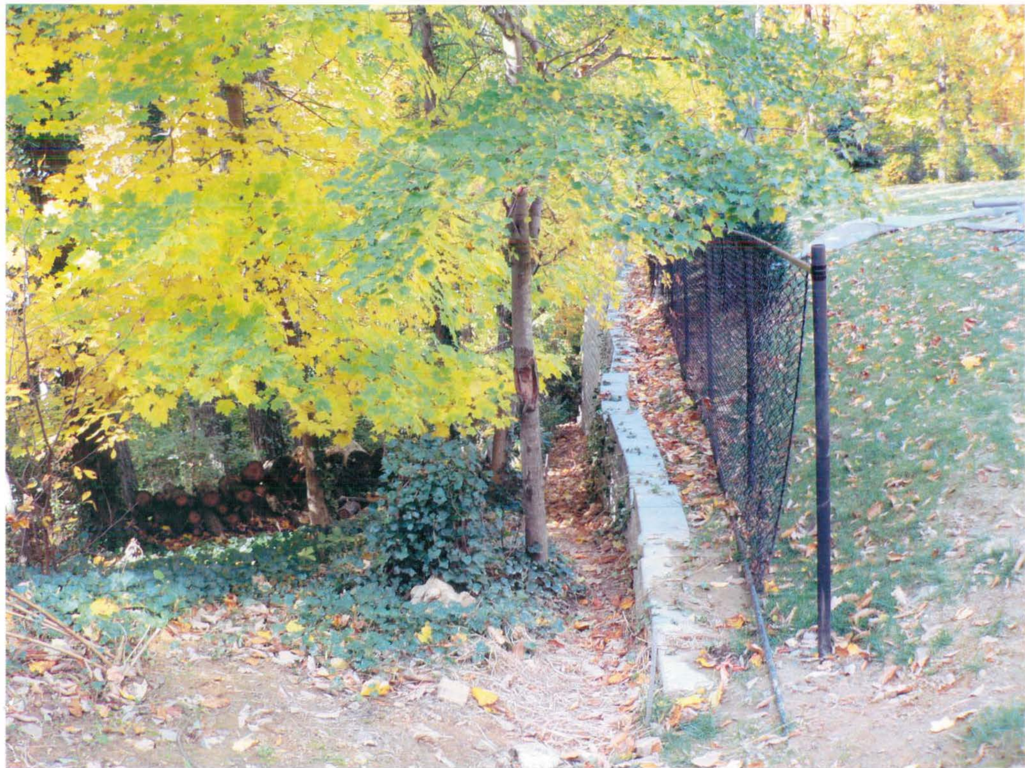
side view of wall
