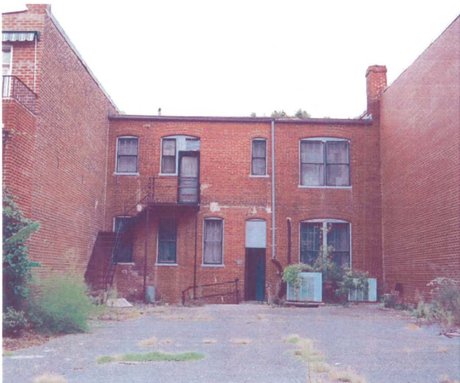
LOOKING AT REAR OF BUILDING
