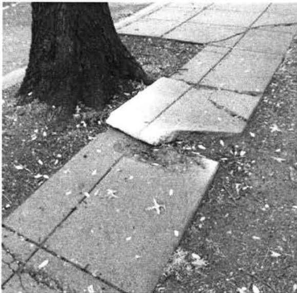
Figure 5: 6 th Street east-side near Gallaudet campus entrance
