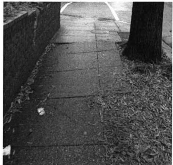
Figure 6: West Virginia Avenue east-side
