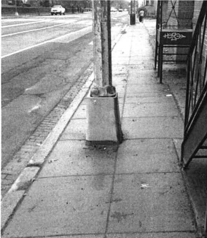
Figure 4: Obstructing Light Fixture along Florida Avenue (south-side between M Street and 7 th Street)
