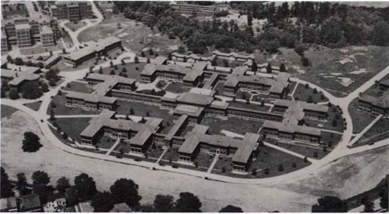
Figure 3.84: An early aerial view of the CT Village.
