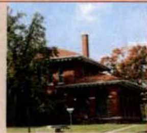
Red brick exterior walls
