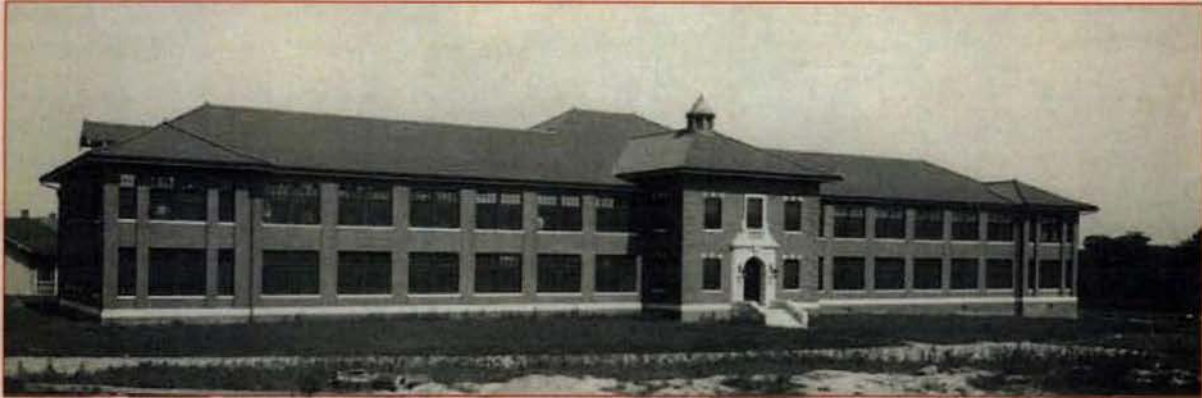
Figure 3.64: A 1932 Picture of Building 102
