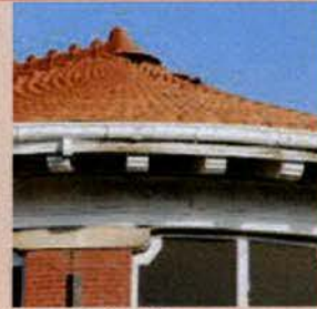
Complex Roof Forms
