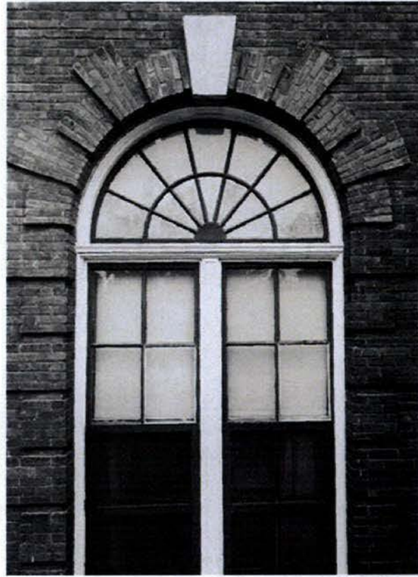
Figure 3.2: Architectural detail of historic Saint Elizabeths
