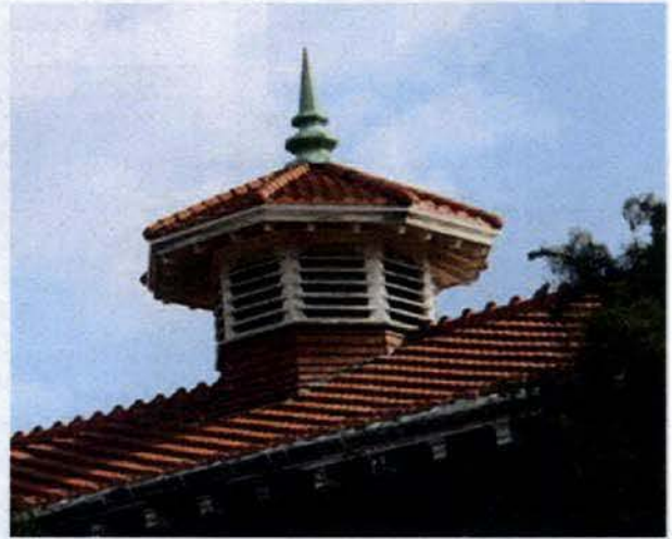
Figure 3.9: . Cupolas are unique to several historic structures.
