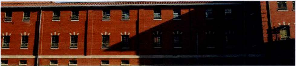
Figure 3.10: Façade ordering in the CT Village group.
