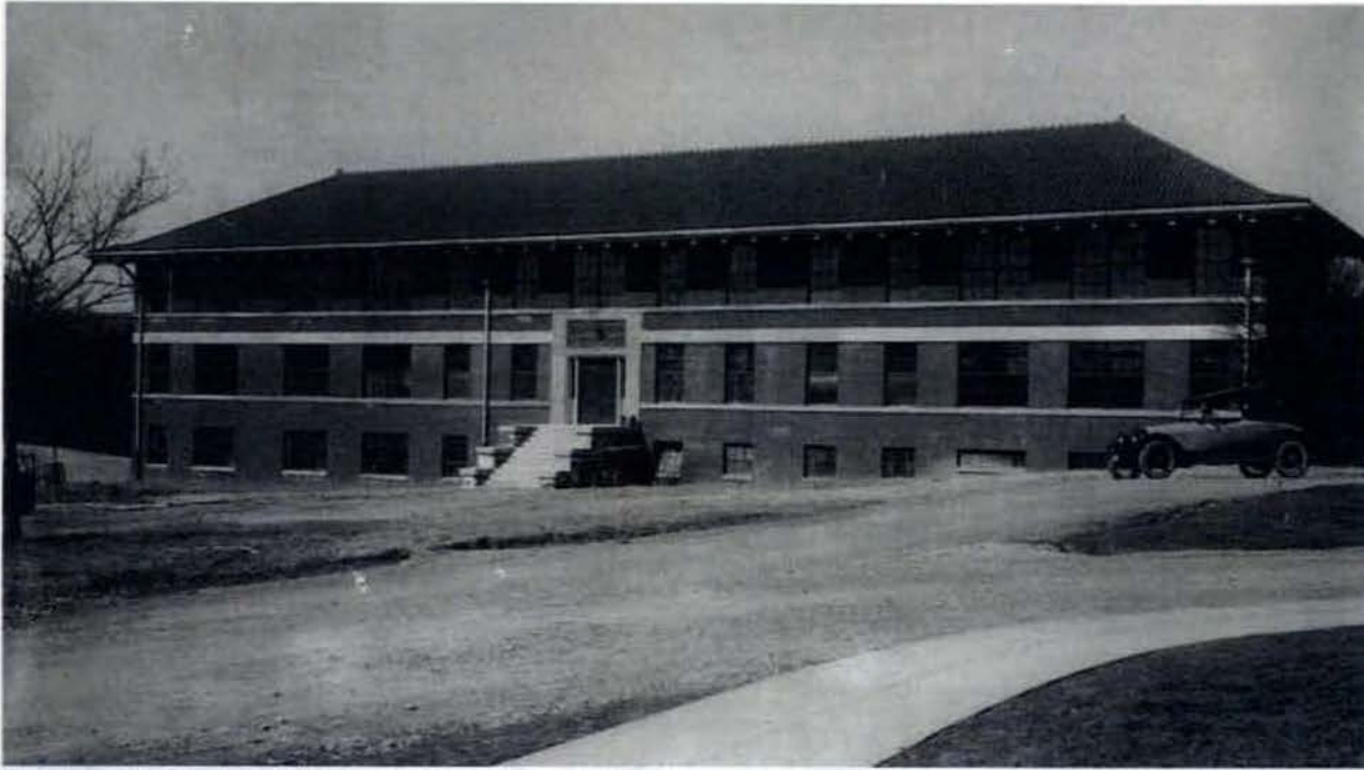
Figure 2.10: Building 88 - Blackburn Laboratory
