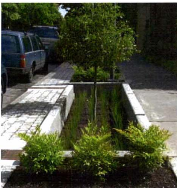
Figure 2.31: Tree pits can be designed to collect stormwater.
