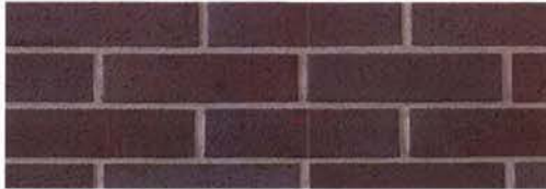
BRICK 2 - WEST BUILDING
