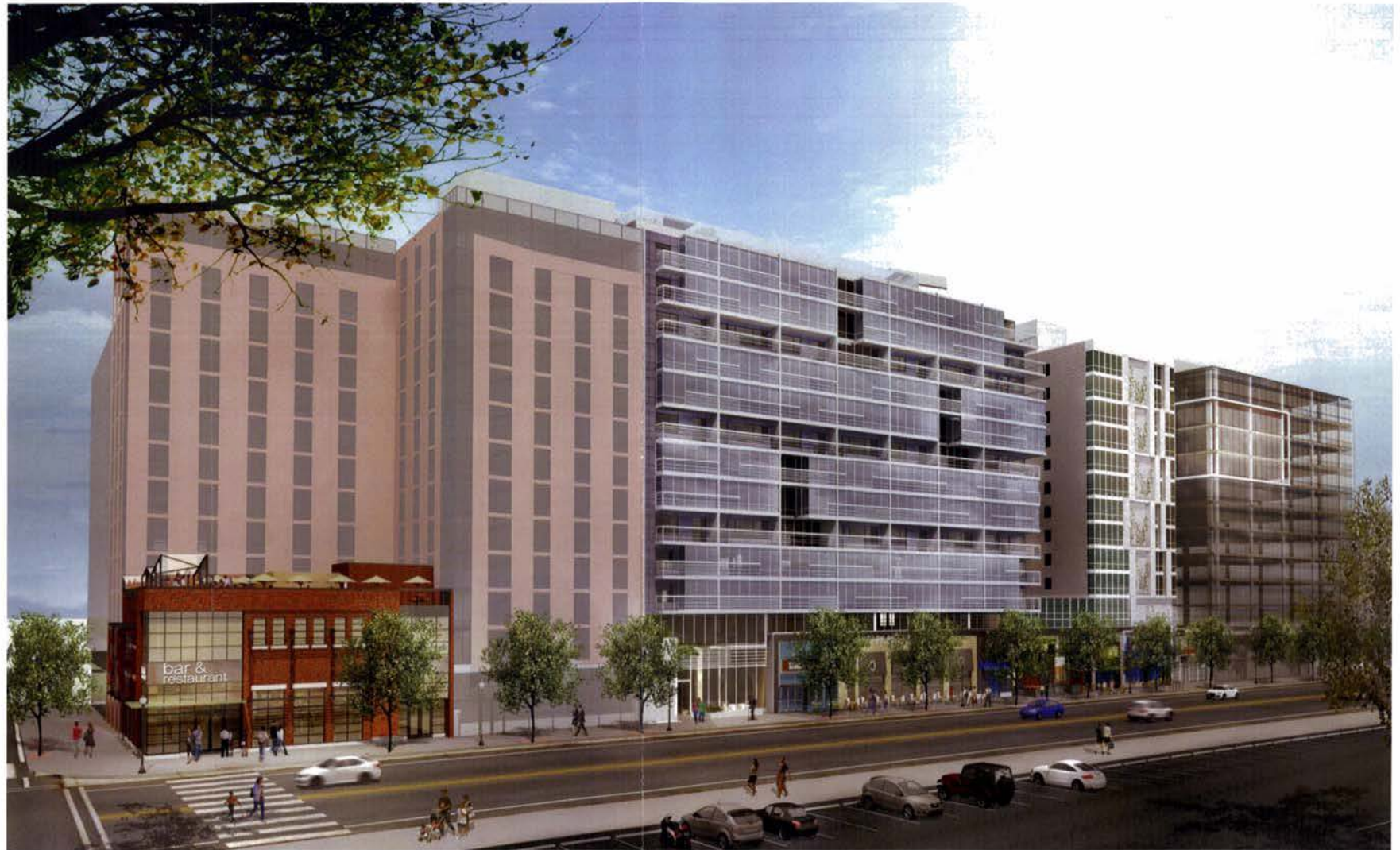
VIEW OF FIRST STREET SE
