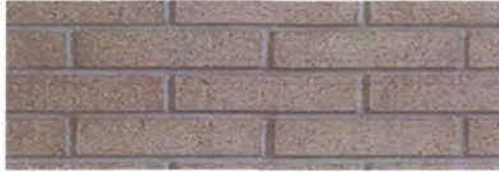
BRICK 1 - EAST BUILDING AND SAWTOOTH BAYS
