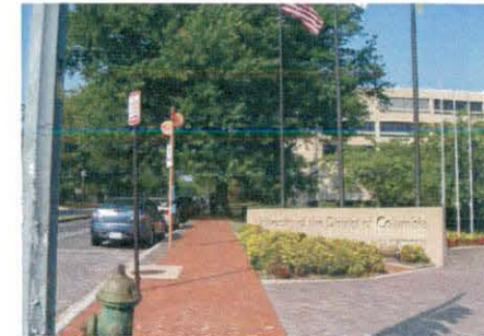
EXISTING BRICK PAVING ON VAN NESS STREET
