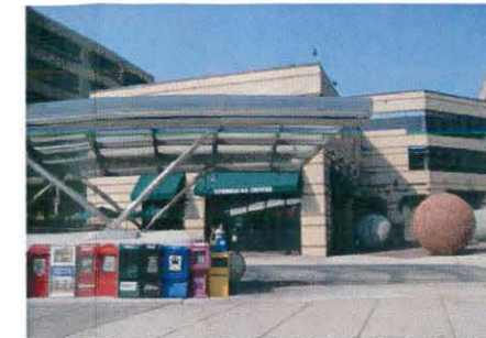
EXISTING CONCRETE PAVING BY VAN NESS METRO STATION
