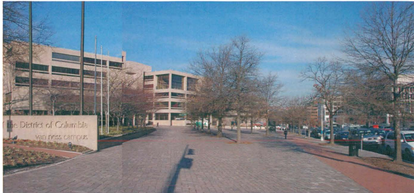
EXISTING PLAZA - VIEWING NORTH
