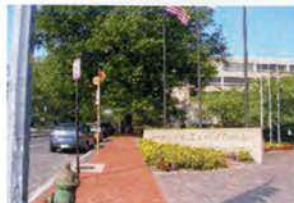
EXISTING BRICK PAVING ON VAN NESS STREET
