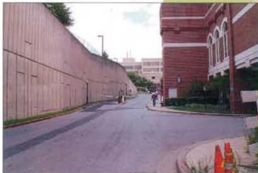
Image 2: Looking north along West Road toward Lombardi Circle: Shows location of Leavey building, Leavey loading area, narrow sidewalks along the east side, roadway conditions, traffic gate location, lack of sidewalks along west side and grade change/retaining wall to the west.
