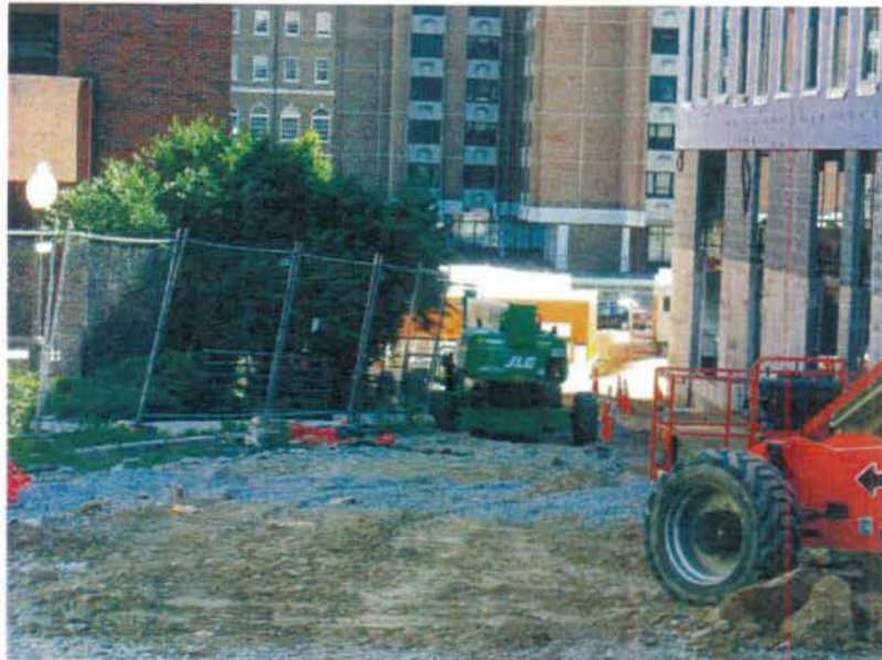
Tondorf Road looking south. This portion excavated during construction of the New Science Building can be replaced.
