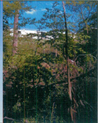
The white structure is a retaining wall, built after the 2010 collapse of the slope.
