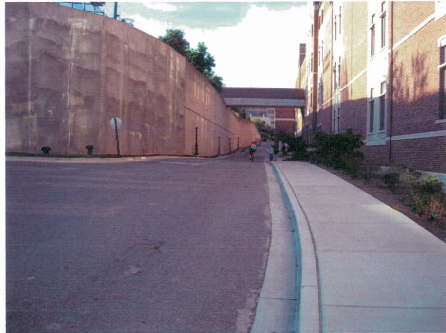
Kehoe Field retaining wall on left, business school on right. Note pedestrian bridge overhead in the distance.
