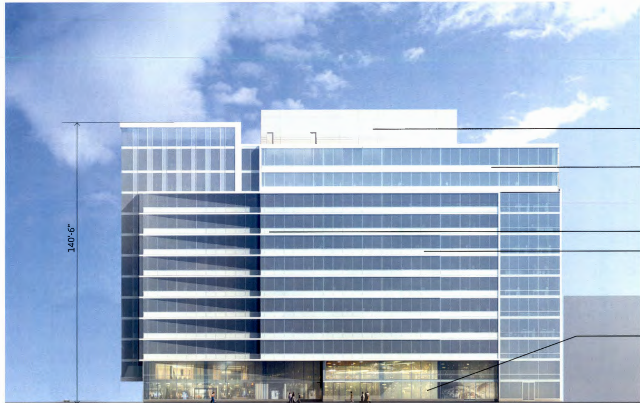
Precast Concrete Penthouse Enclosure
