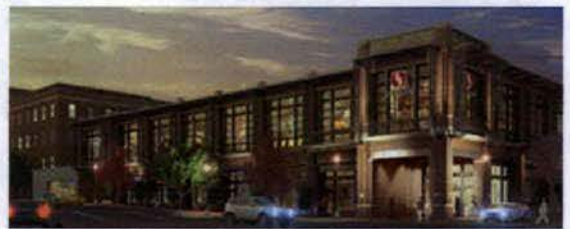
Georgetown Safeway, Under Construction
