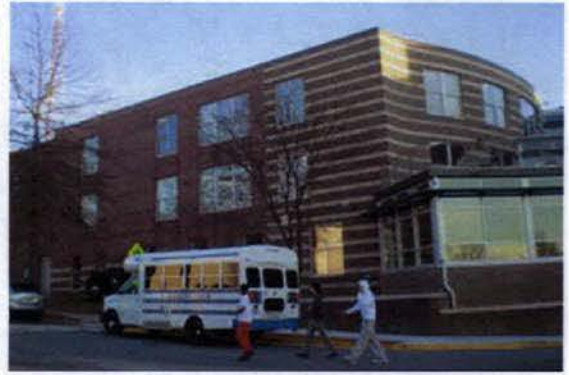
Georgetown Day School, Davenport Street Elevation facing Safeway Showing existing flush masonry banding along Davenport Street.
