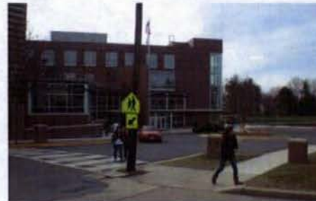
6 - View of Georgetown Day School from existing Safeway Parking lot
