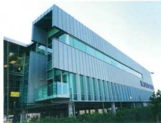
STANDING SEAM METAL PANEL
