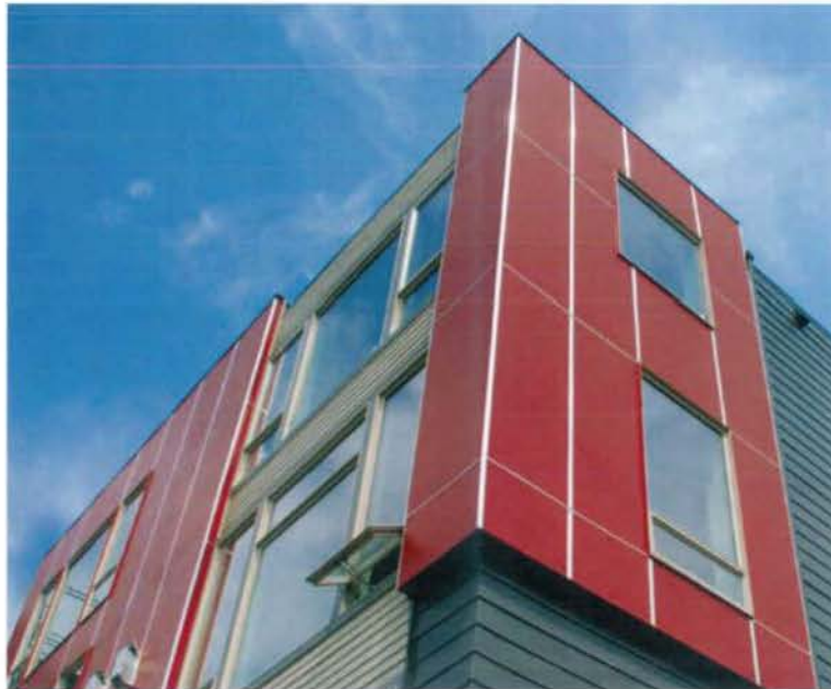
HARDIE PANEL SIDING WITH METAL REVEALS
