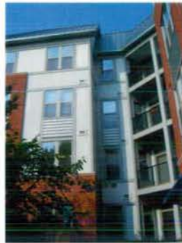
HARDIE PANEL SIDING WITH BATTENS
