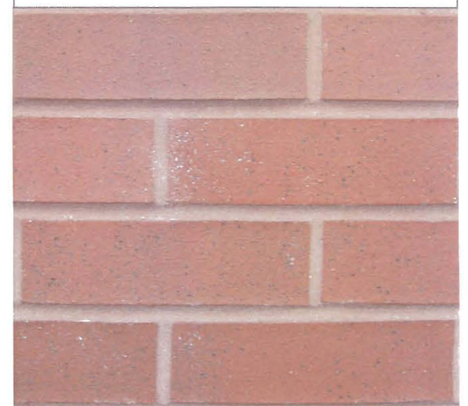
Buildings A3 & B2 - Main Brick
