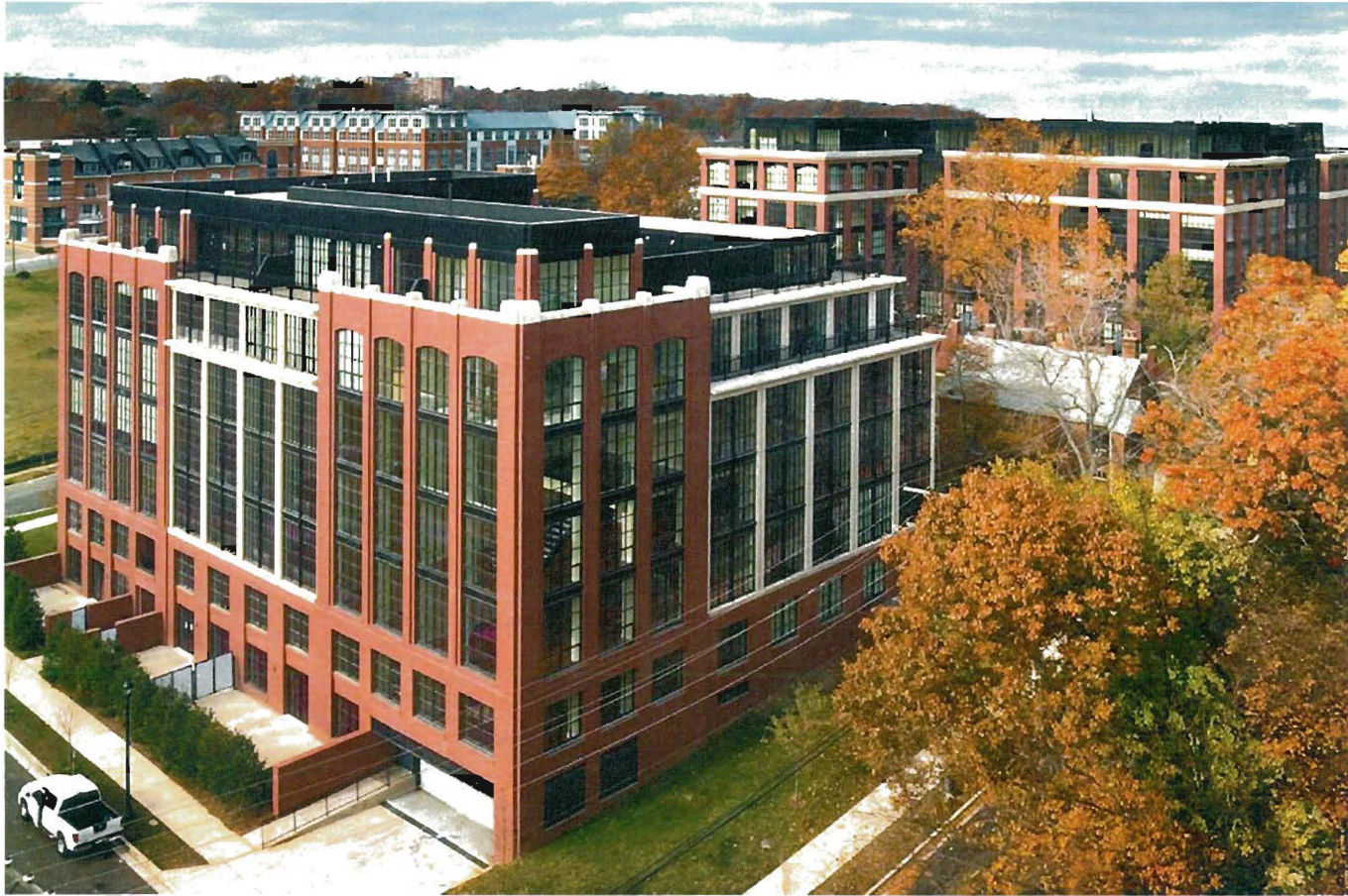
The Mercer Lofts
