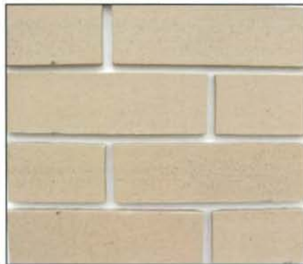
Building A1 - Main Brick
