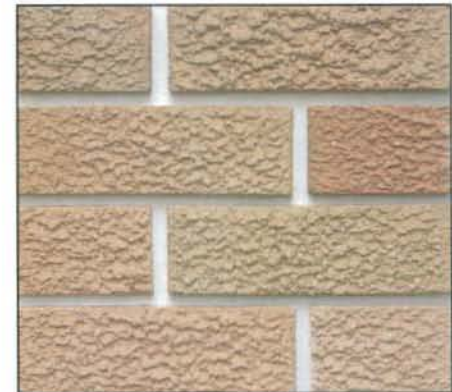
Buildings C3 - Main Brick
