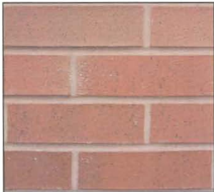
Building A3 and B3 Brick
