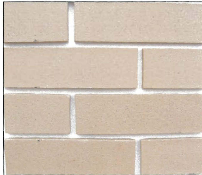
Building A1 - Main Brick
