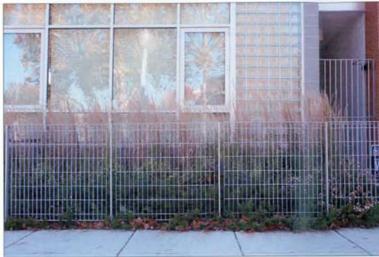
IMAGE OF FENCE AT 442-444 N STREET, NW SHOWING TRANSPARENCY OF MATERIAL AGAINST VEGETATION
