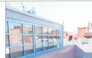
EXAMPLE OF CORRUGATED SIDING (626 S STREET, NW)
