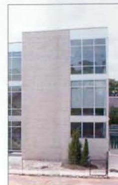
EXAMPLE OF ARCHITECTURAL CMU & ALUMINUM WINDOWS (506 O STREET, NW)
