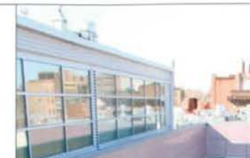
EXAMPLE OF CORRUGATED SIDING (626 S STREET, NW)
