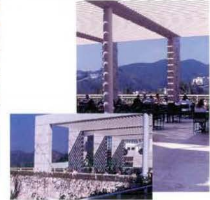
Screen Structure at Restaurant
