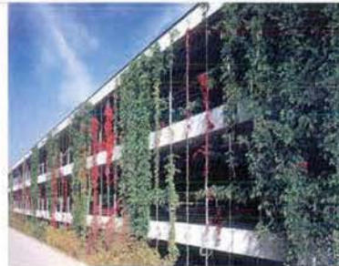
SUPPORTING SYSTEM I: CLIMBING PLANTS TRAINING SYSTEM AT- TACHED THROUGH WALL MOUNTING COM- PONENTS, WHICH MAINLY INCLUDES STEEL ROPE, HORIZONTAL RODS, AND SECTION CONNECTORS
