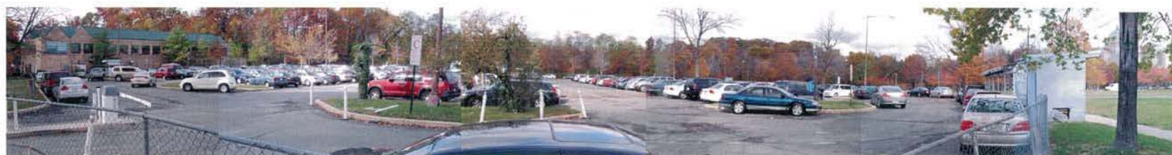
3 View of site from Michigan Ave.
