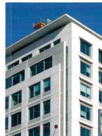
ARCHITECTURAL PRECAST TYPE I ACID ETCHED FINISH
