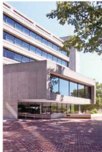
BOARD ROOM FROM PLAZA
