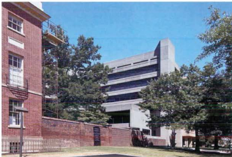
FRONTAGE ALONG NEW YORK AVENUE
