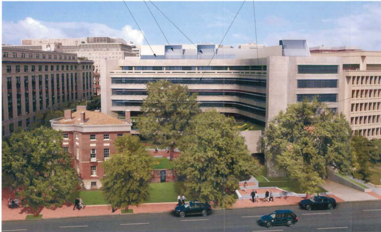
AIA HEADQUARTERS AND OCTAGON FROM NEW YORK AVENUE
