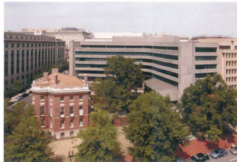
AIA HEADQUARTERS AND OCTAGON FROM NEW YORK AVENUE
