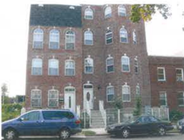
② LAMONT ST. - VIEW SOUTH
