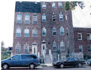
② LAMONT ST. - VIEW SOUTH
