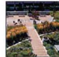
PHOTOS OF GREEN ROOF
