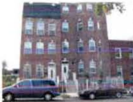
② LAMONT ST. - VIEW SOUTH
