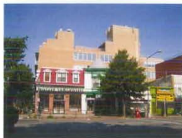
④ GEORGIA AVE. - VIEW WEST
