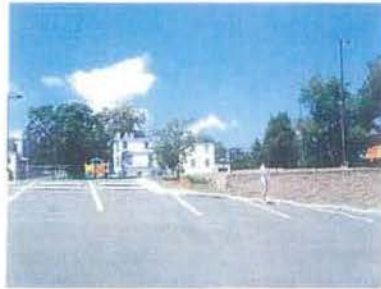
EXISTING PARKING, RETAINING WALL
