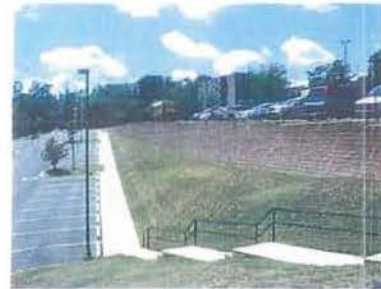
EXISTING RETAINING WALL
