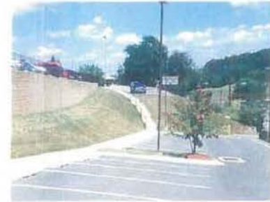
EXISTING RETAINING WALL
