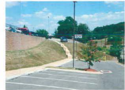
EXISTING RETAINING WALL
