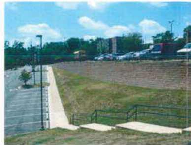
EXISTING RETAINING WALL
