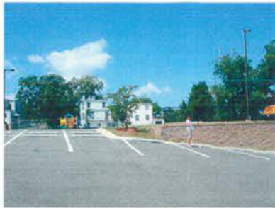
EXISTING PARKING, RETAINING WALL
