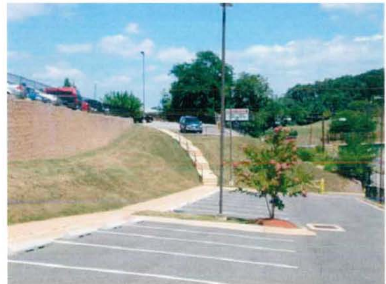
EXISTING RETAINING WALL
