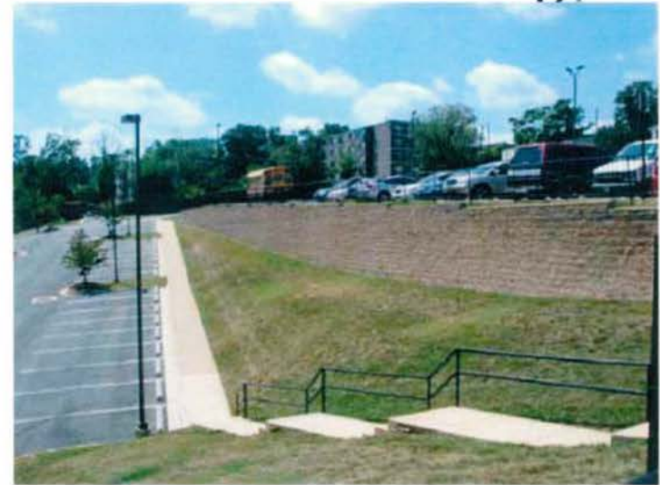
EXISTING RETAINING WALL
