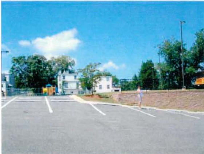
EXISTING PARKING, RETAINING WALL
