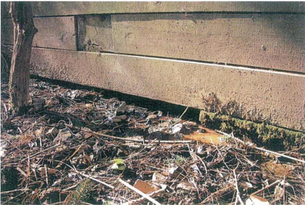
Photograph 4: Additional picture of groundwater seep/ spring originating from existing Canal View retaining wall.
