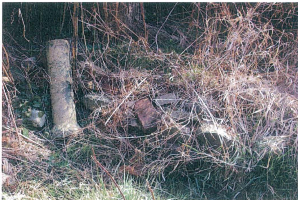
Photograph 1: Existing groundwater seep/ spring near the end of Lingan Way.
