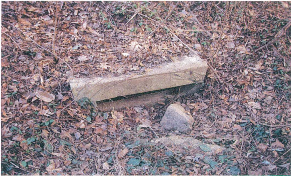
Photograph 5: Existing drain inlet near Riverside Hospital exercise area in the northwest portion of the property.
